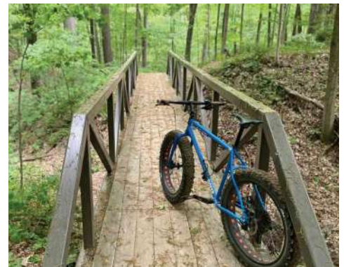
Allegan Mountain Bike Trail truss bridge, courtesy of Tom Slocum, 2025.
